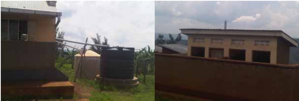
Figure 9.4: Rainwater harvesting with PVC tanks (left); VIP at Ruhira District health center (right)
