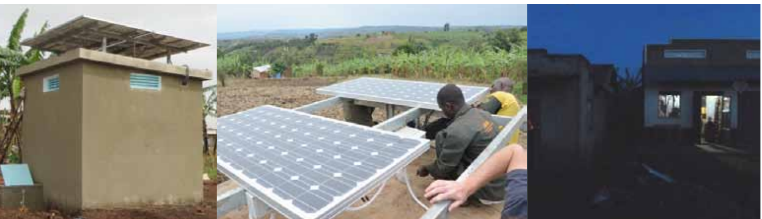
Figure 9.1, SharedSolar, (left to right): a shed housing the batteries and electronics; solar panel installation; home with electric lights powered by SharedSolar next to a home using kerosene lighting
