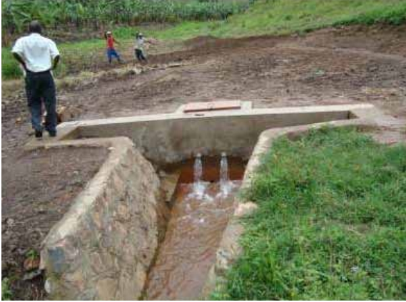
Figure 9.9: Protection of Ruhiira's water source
