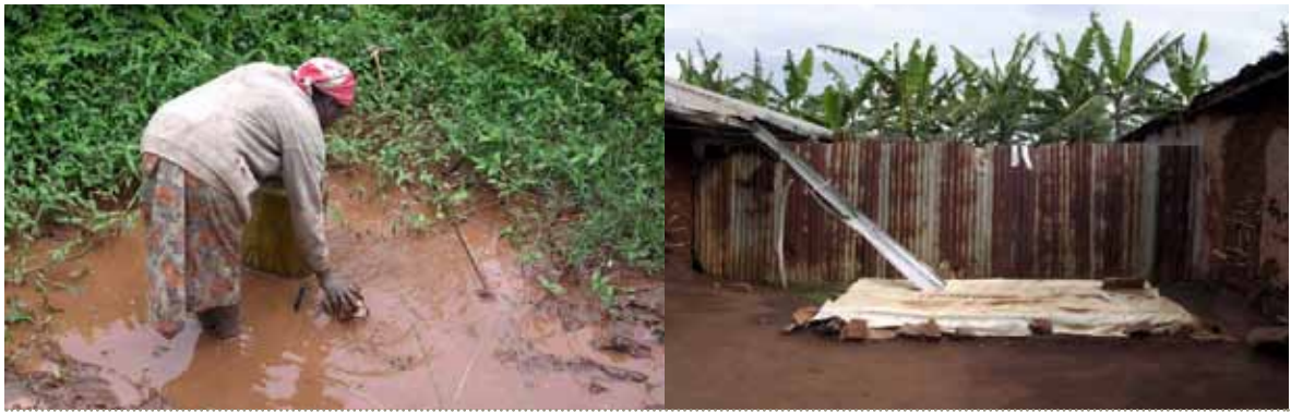
Figure 9.7: Collecting water from a ditch (left); rainwater harvesting from roof to underground tank (right)
