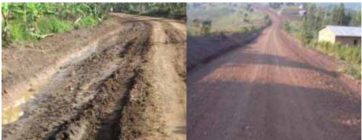
Figure 9.6: Rehabilitation of the Kaaro-Karungi-Kisyoro road, before (left) and after (right).
