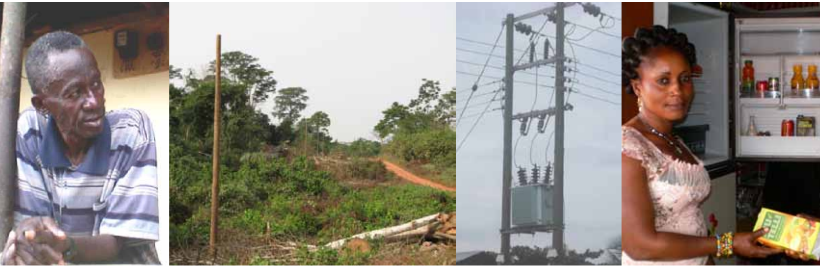
Figure 6.3 (left to right): A customer with a new meter; clearing trees for grid construction; a transformer in Dawusasoo; a Datano business using refrigeration.
